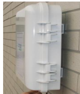
FDB fiber termination box on the wall
